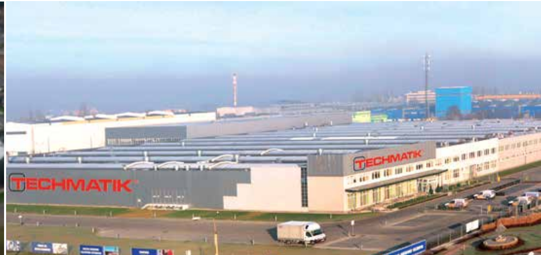
Techmatik Facility - Radom, Poland
